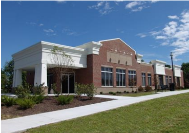
Medical Office Building, Union, KY
