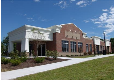
Medical Office Building, Union, KY
